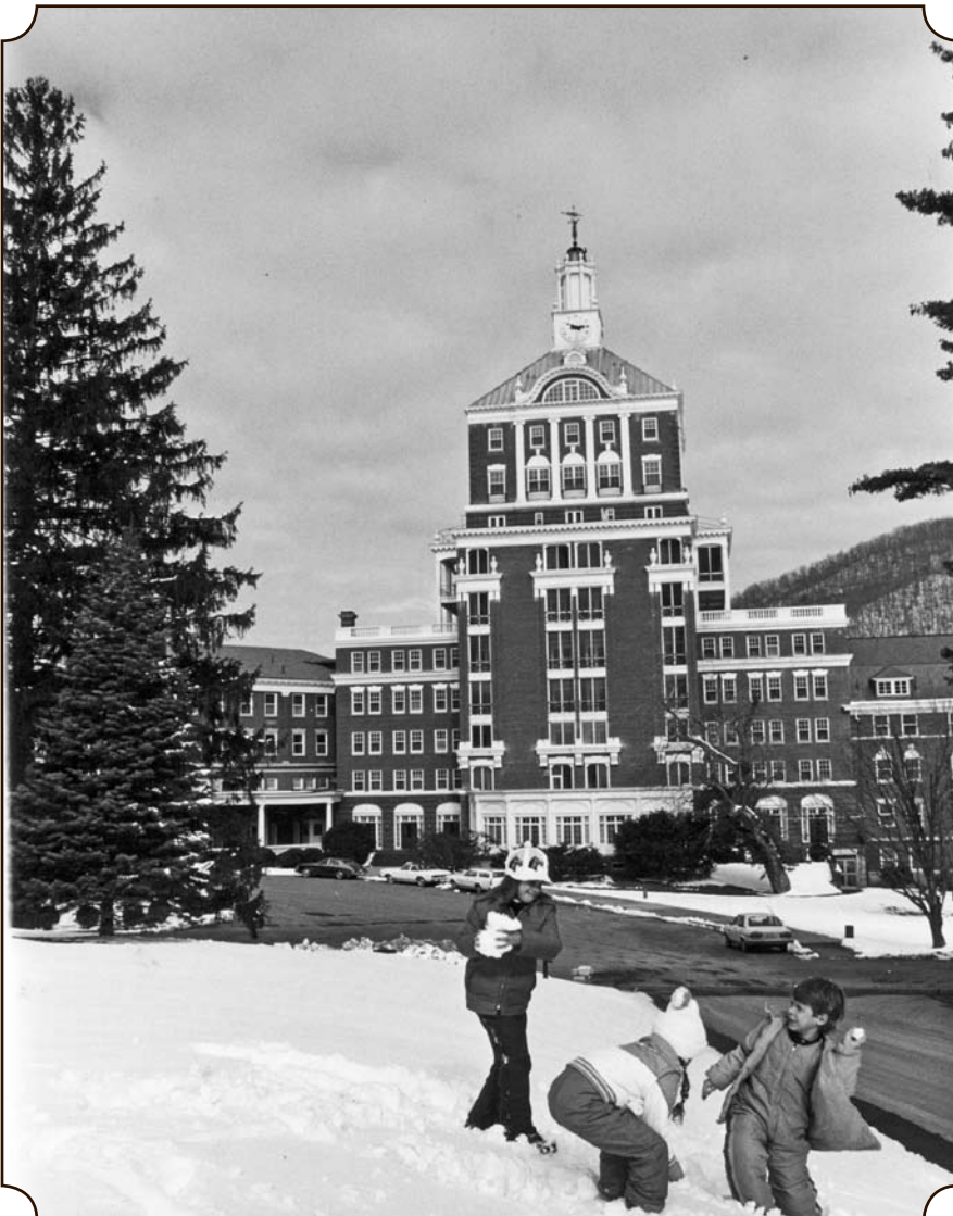
Top; Clearing the slopes at The Homestead in 1959. Bottom; The towering edifice of The Homestead. Pulling up out front is a passport to a luxury dining and lodging experience.
